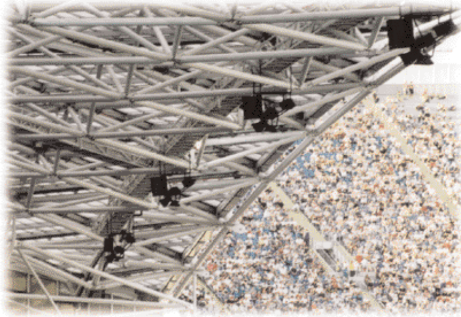
The leading edge of the roof of both the East and West Stands is above the front row of the seating, which provides an ideal position for the seven-speaker clusters. Photo: Brian Chilcott.
